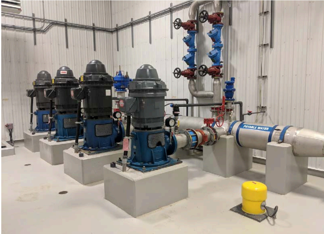
Treated Water pumps that feed our transmission mains and City of Brooks water distribution network.
