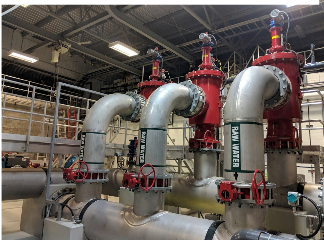
Raw water piping that feed the membranes
